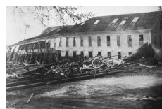
Damage to a building in Bristol. - Courtesy NOAA
